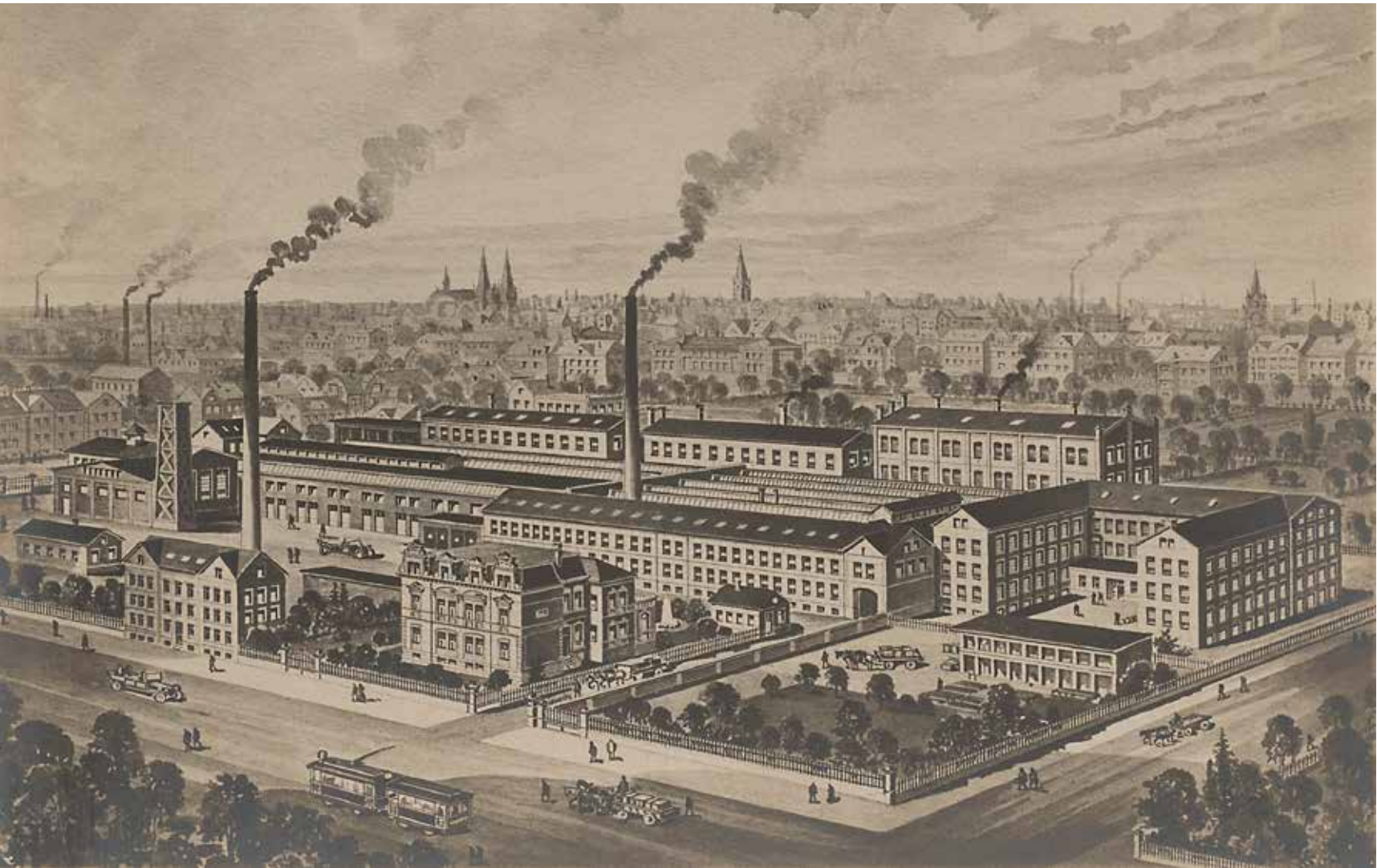
| As was typical at the time, twice as many windows are shown in the picture as there actually were. This meant that the windows at the back of the building could also be depicted.
