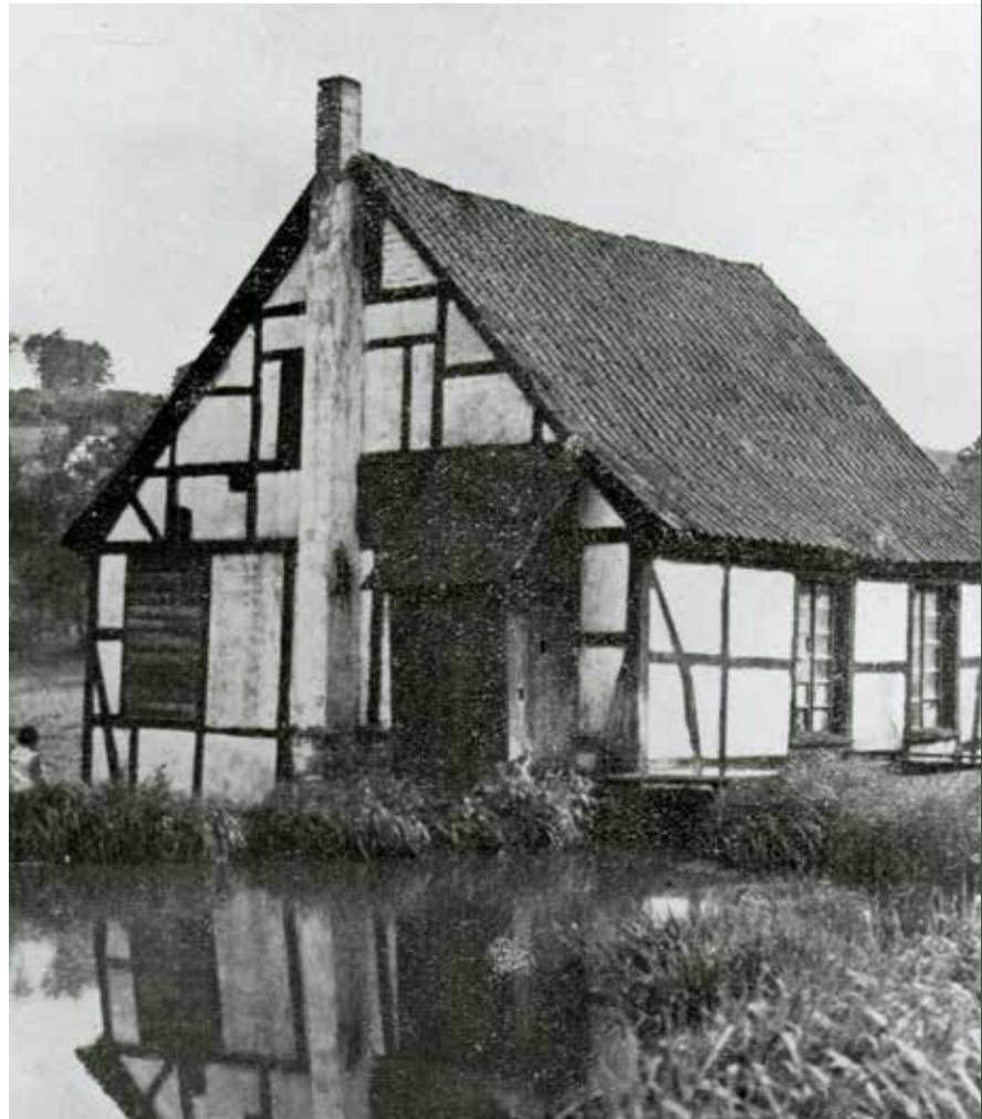
| WÜSTHOF's "Kotten" in the "Weinsbergtal"
