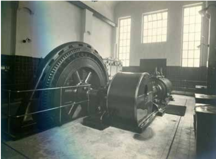
| The newly installed steam engine
